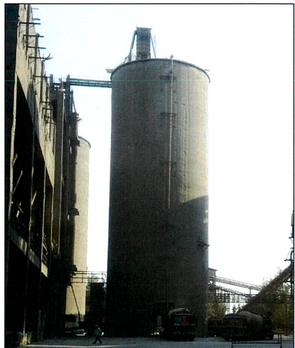
LINE 2 Fly Ash Silo
