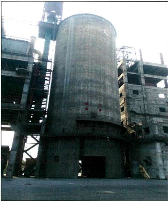
LINE 3 Cement Silo
