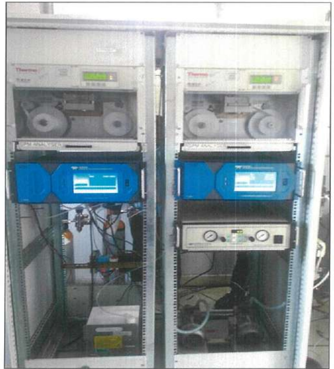
LINE-3 COOLER STACK MONITOR
